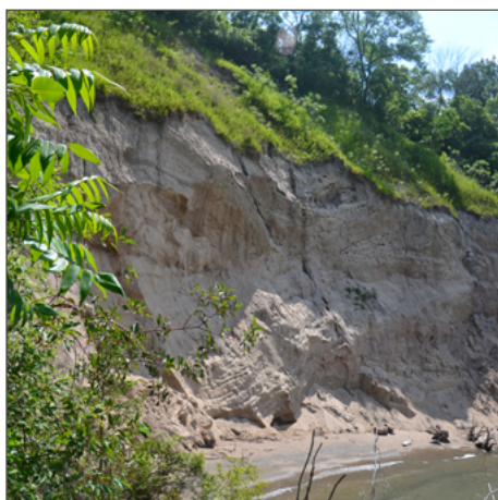
Severe Toe Erosion
