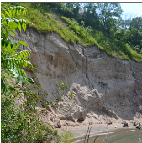
Severe Toe Erosion
